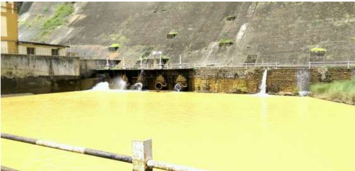
Bhatghar Hydro Power Station
